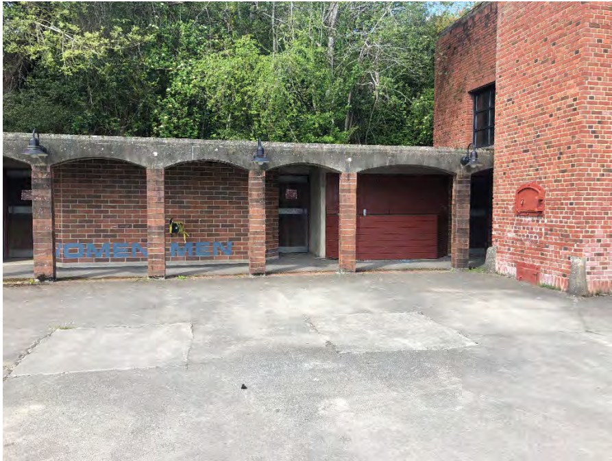
Photograph 6. Existing restroom annex building (April 2021).
